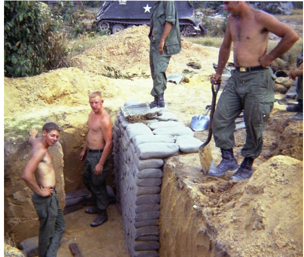
Dau Tieng bunker building
